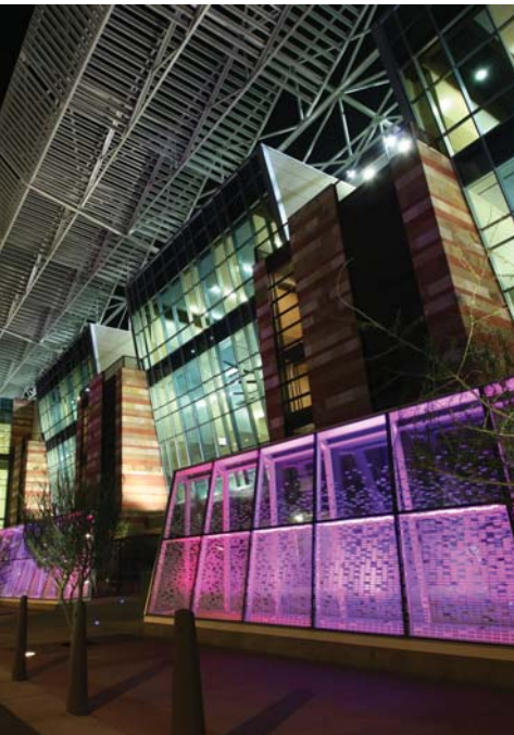
Lighting Crystals - North Building
